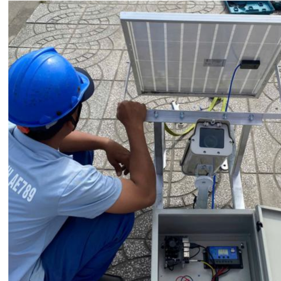
AI CCTV system installation – Can Tho, Vietnam
